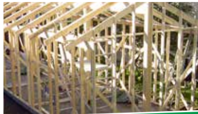
JOISTS FOR THE FRAMEWORK
