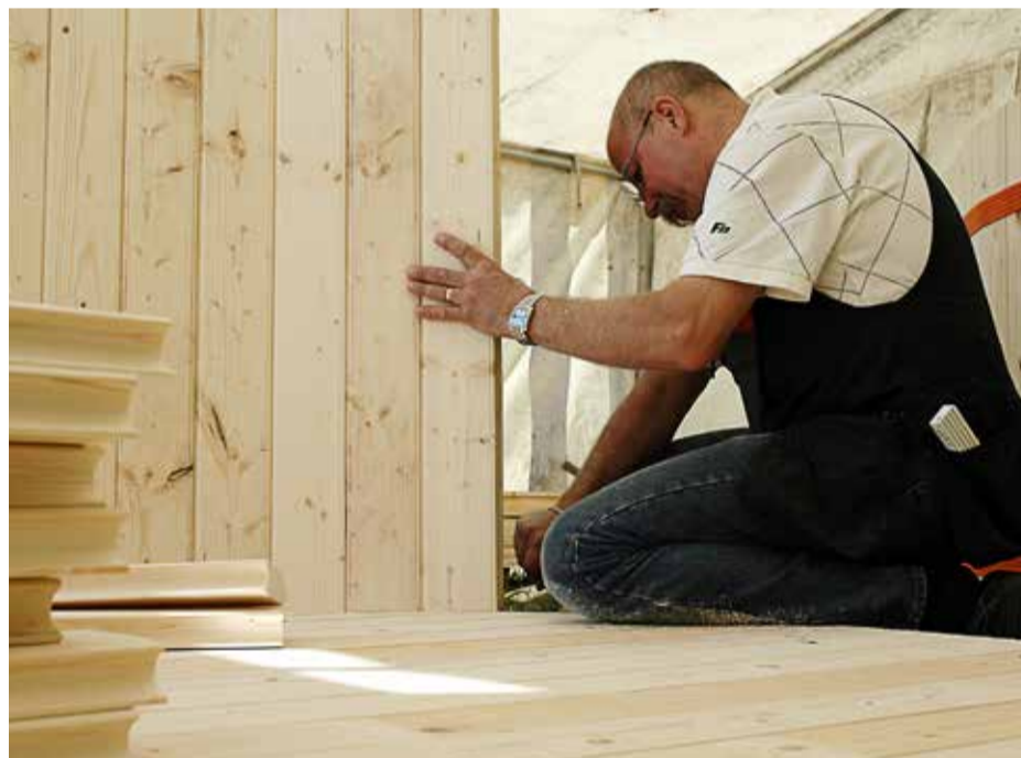
Take a LOGOSOL training course and build your own outdoor hot tub – and take it home with you.
