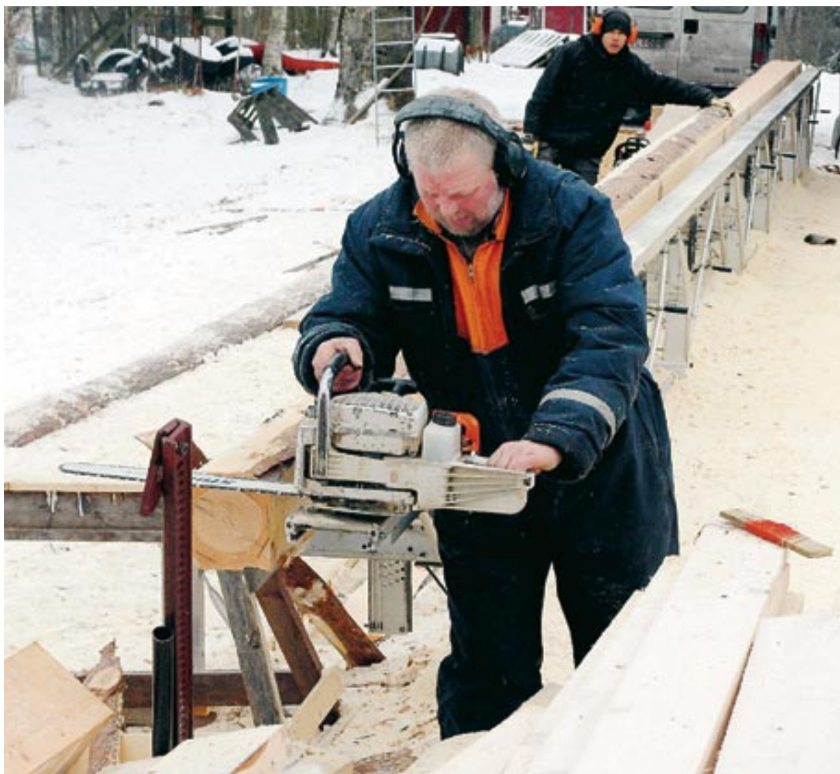
Poul Niensens three and a half M7s were the only way that the 17-metre long, ruler straight beams could be cut out for use in rebuilding the church tower in Vadensjö.
