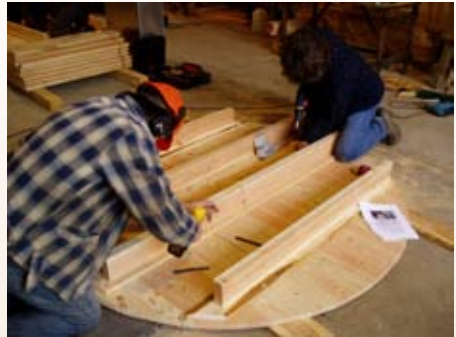
The T-beams are screwed to the bottom.
