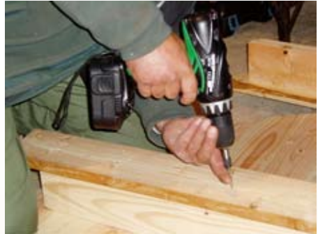
The T-beams are screwed together.
