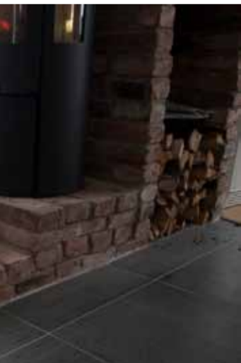
• The stairs are made of recycled bricks from an old chimney.
