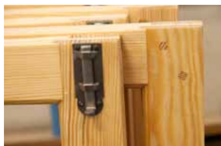
• The window frames are put together with wood dowels to make it easier to replaced damaged details in the future.
